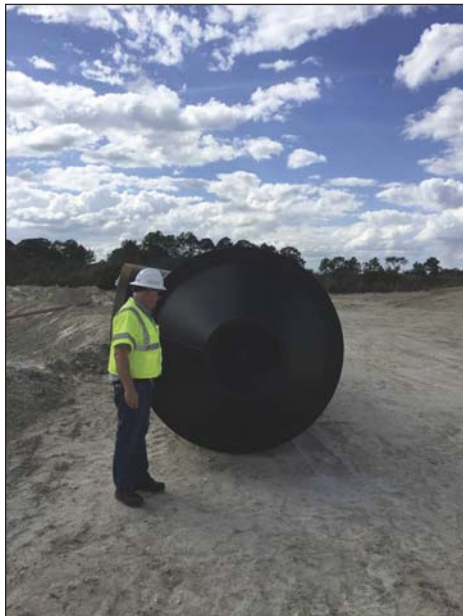
Photo 3. S472 Pump Can
