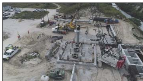
Photo 5. S476 Pump Can Installation
